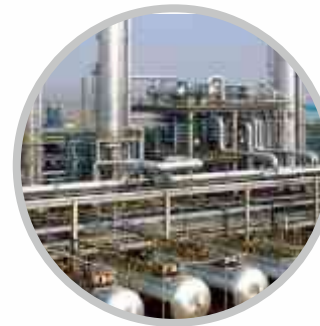
Processing Plant Refinery
